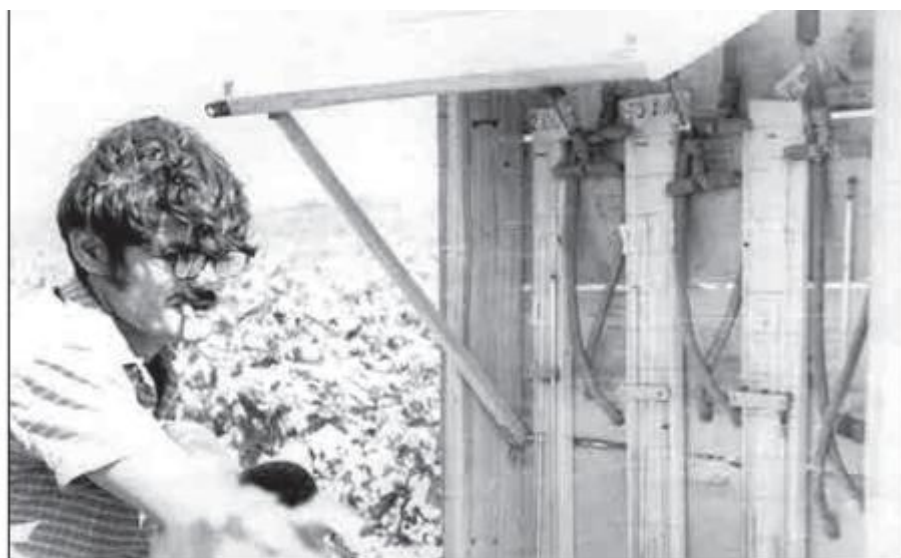
Figure 1. Measurement stand with mercury vacuum gauges in field conditions on soils of Agricultural Site No. 11 of the Karshi Steppe.
