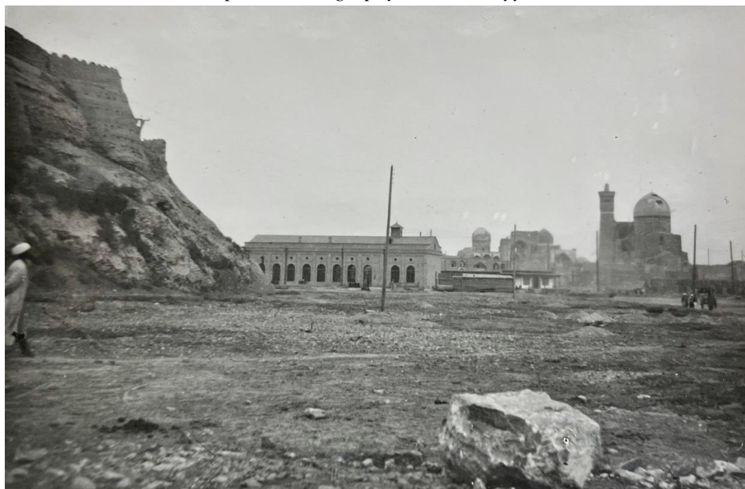
Figure 8. The first diesel power plant building built on the site of the lower courtyard Palace 1924 y.
