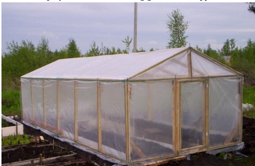
Figure 4. It is a greenhouse with wooden structure with transparent film.
