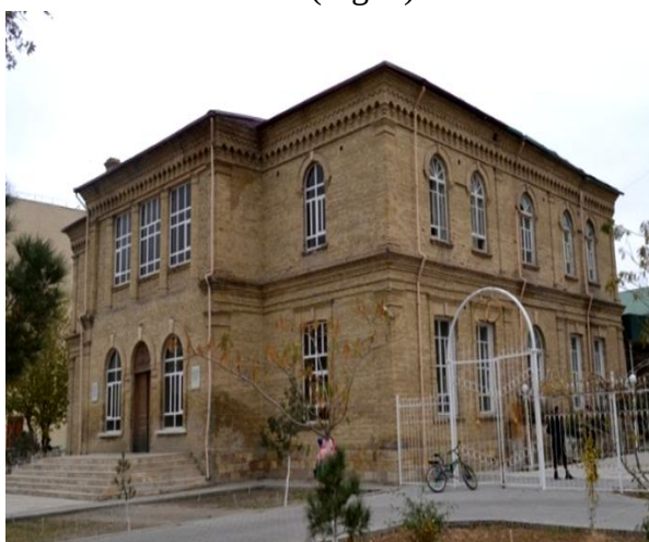
Fig. 4. General view of the "House of Scientists" building (from the northwest)
