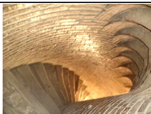
Fig. 2. A fragment of the interior walls and staircase of the Kalyan Minaret, made of baked brick.
