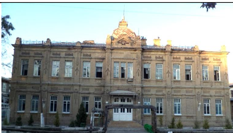
Fig. 11. General view of the building of the current administration of the regional multidisciplinary medical center.
