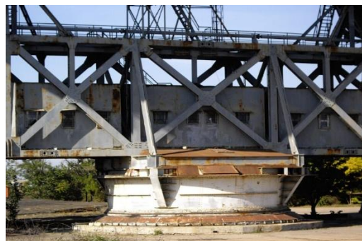
Figure3. Railway bridge truss
