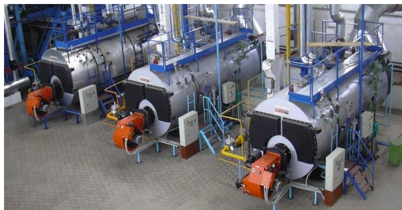
Fig.1. Water treatment for boiler plants
