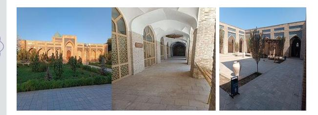
The sides of the Odina mosque were built in the proportion of 50x40 meters. The places of worship inside the mosque are wide, and high, with a small dome on top, and thick brick columns are connected to each other through vaults. There is a large mihrab on the west side of the mosque. The prayer "Ayatal Kursi" from the Holy Quran is written in golden letters around the arch. There are seven marbles, on the right side of the mihrab, on which the sermon was read during the Friday and Eid prayers.
